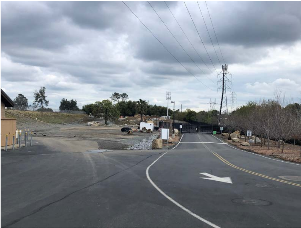
Figure 1 Tank Location - Looking South
