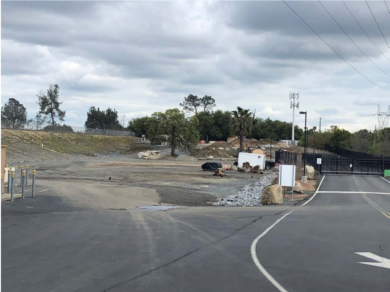
Figure 3 Tank Location - Looking South
