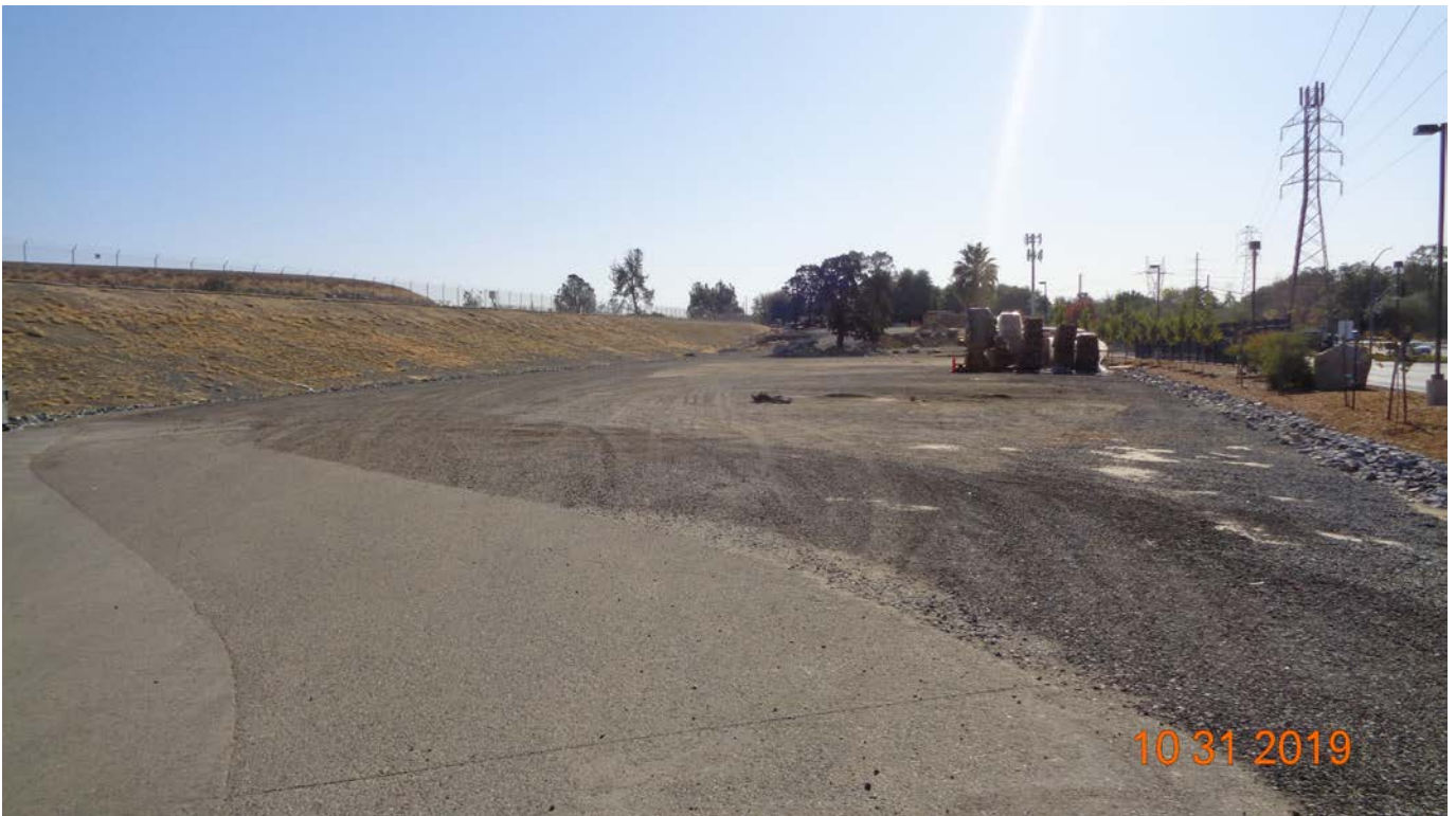
Figure 2 Tank Location - Looking South
