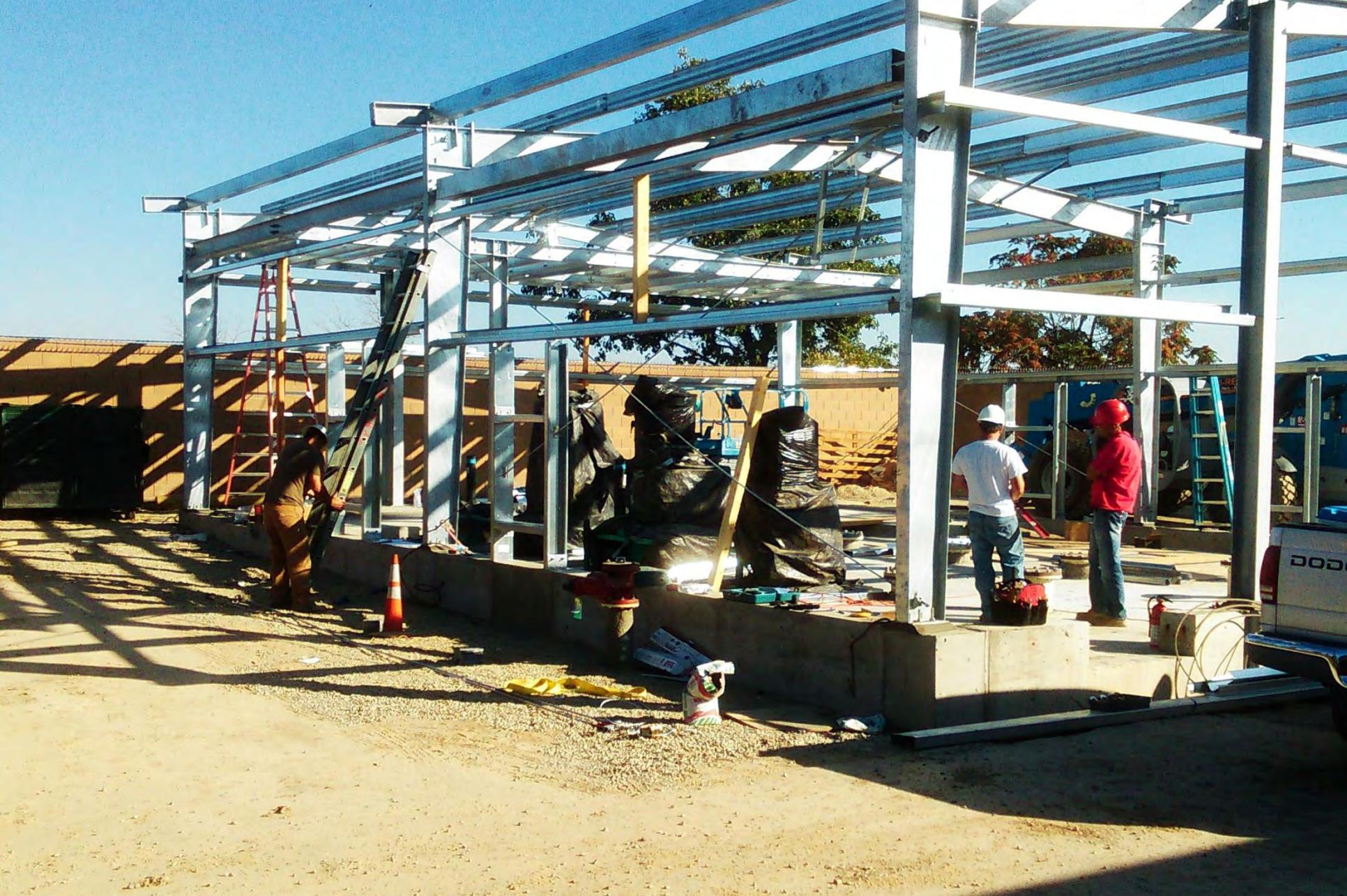
31AM Tie Rod bracing installed; note rod passing through
