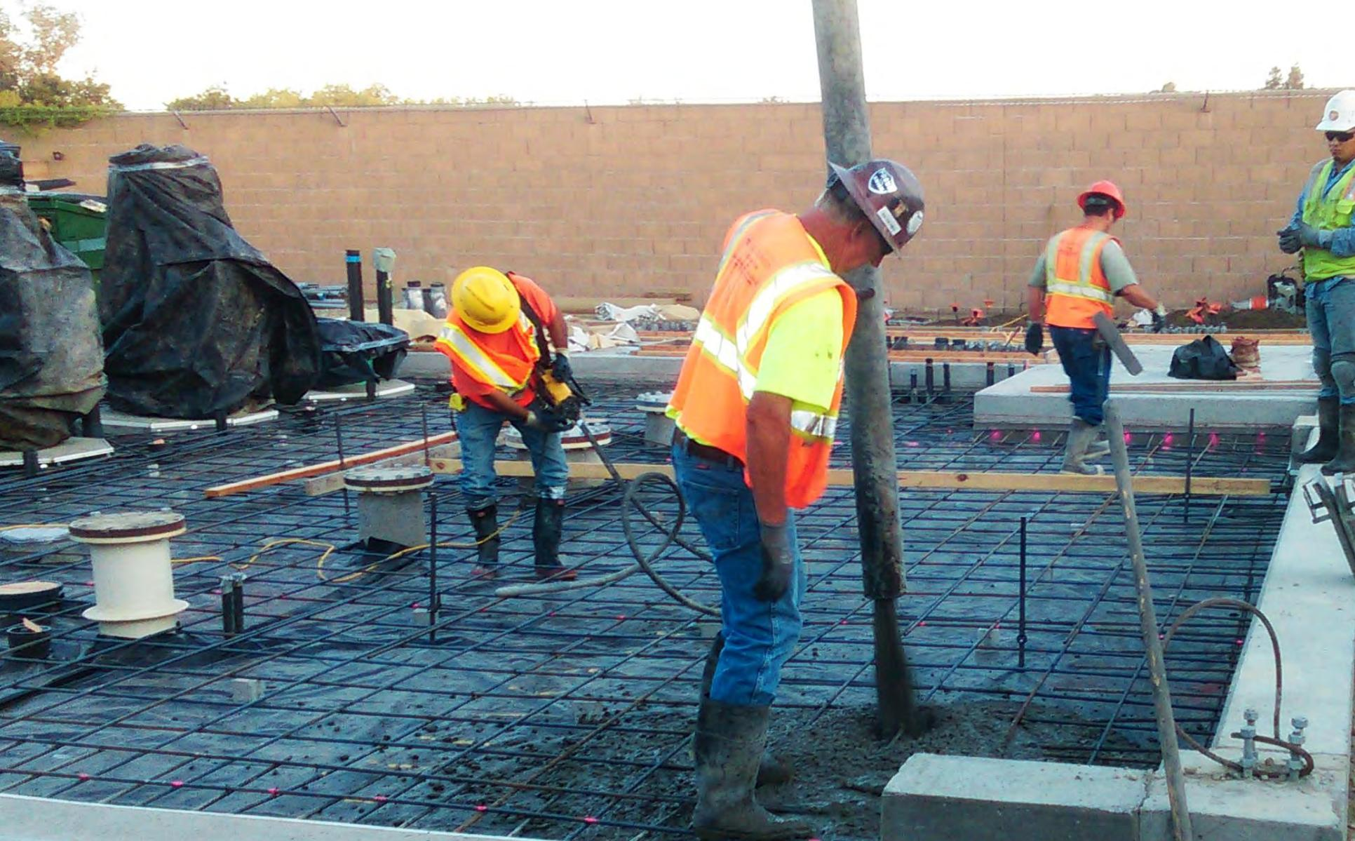
15, 6:09AM A slump sample was taken off the pump
