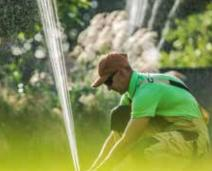
Turn your system on one station at a time. Check for broken sprinklers or leaks and make replacements where needed.
