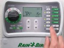
Make sure your irrigation controller battery works. If it doesn't, your controller will go back to its factory settings if power is lost.
