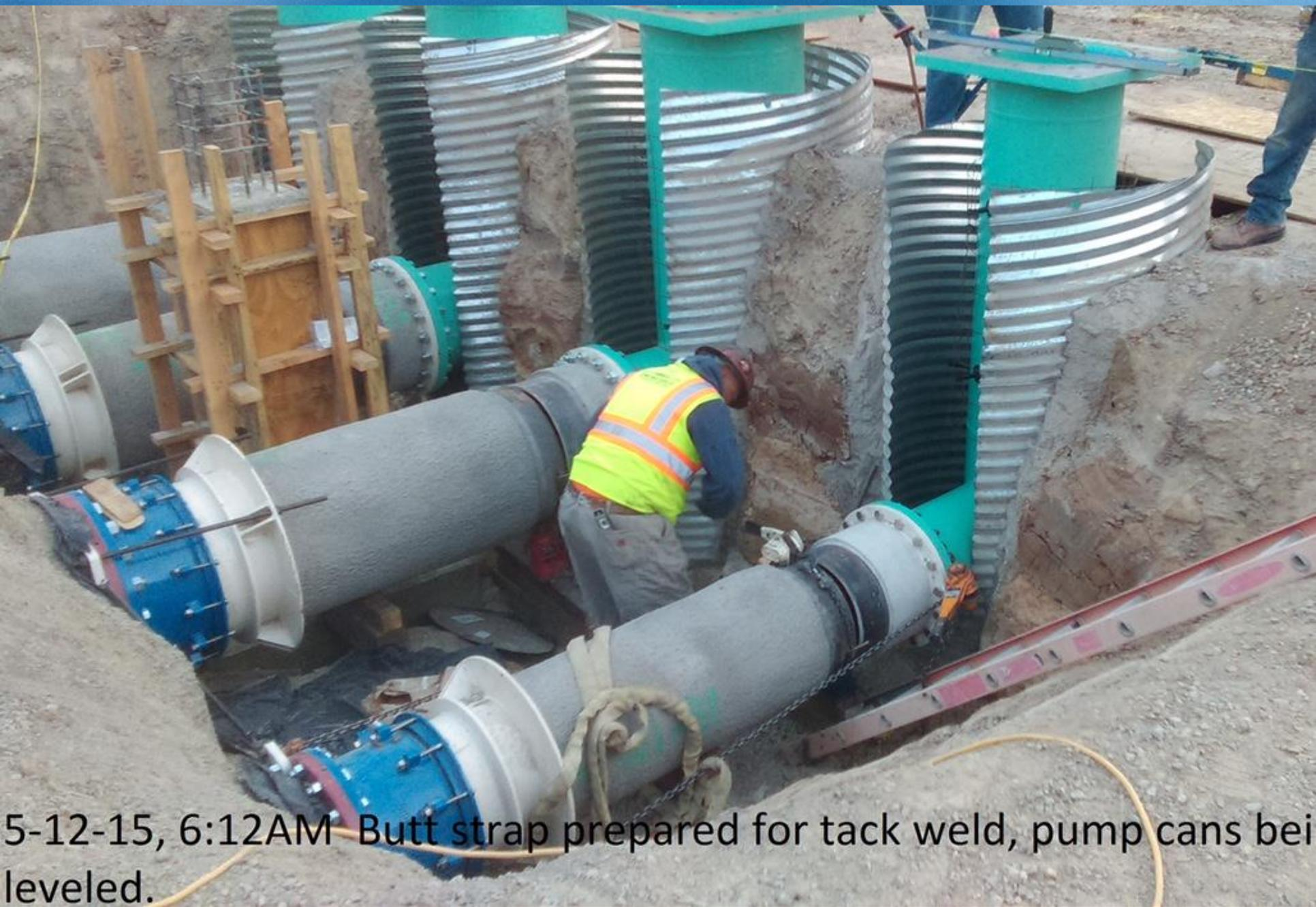
5-12-15, 6:12AM Butt strap prepared for tack weld, pump cans being leveled.
