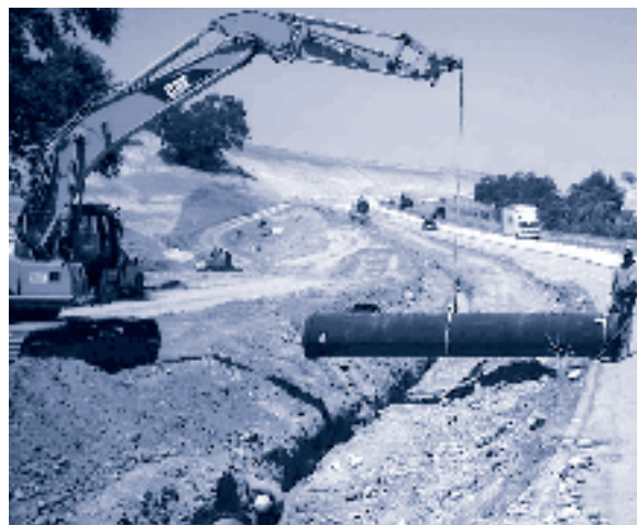
Sierra College Blvd. Water Transmission Main Project
