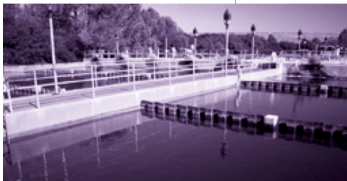
San Juan Water Treatment Plant
