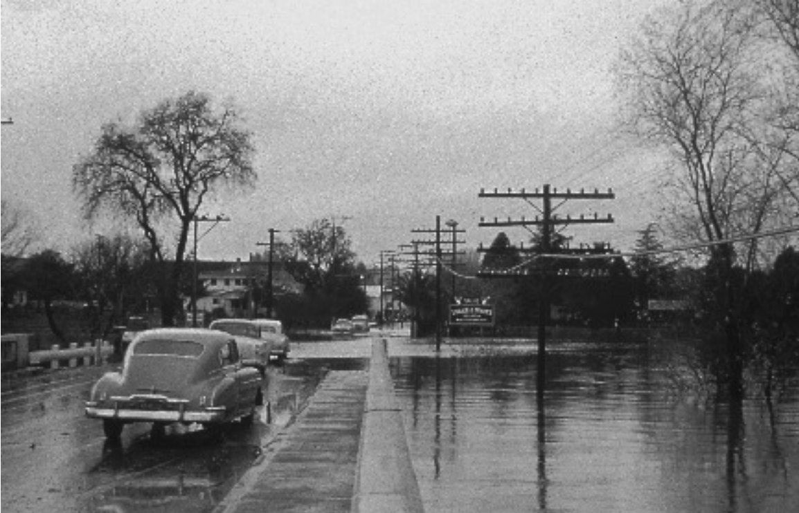
WHEN A MAJOR FLOOD STRUCK IN 1955, SACRAMENTO WAS SPARED SERIOUS DAMAGE THANKS TO THE NEARLY COMPLETED FOLSOM DAM.
