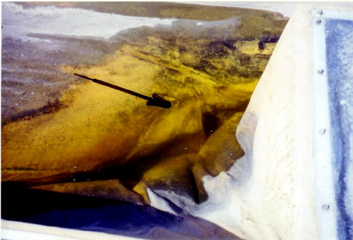
Figure 18. Water Accumulation at Outlet Structure. Note that this Area Contains Numerous Field Seams Due to Structure Attachment.
