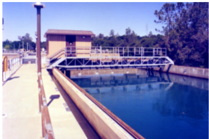
As a critical piece of process equipment, two filter backwash units should be provided in each existing and new filter basin.
