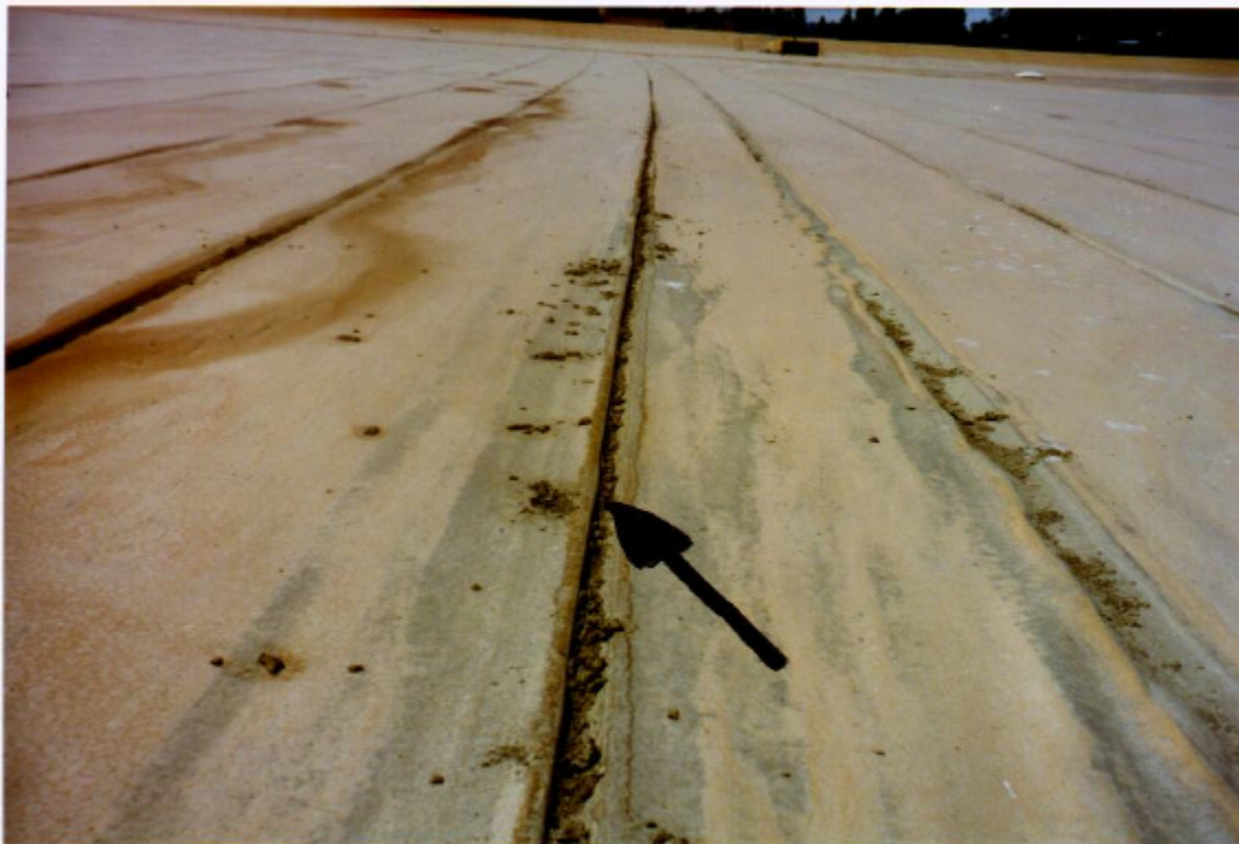
Figure 13. Factory Seam Area Over Water with Accumulated Debris in Channel. Note that Channel Appears to be a Seam Distortion over Water Only.
