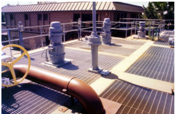
The existing instantaneous blending pump (background) and rapid mix pumps (foreground) should be replaced with a pump jet-injection mixing system for better performance.
