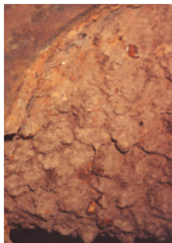
Deposits on inside of Gate Valve
