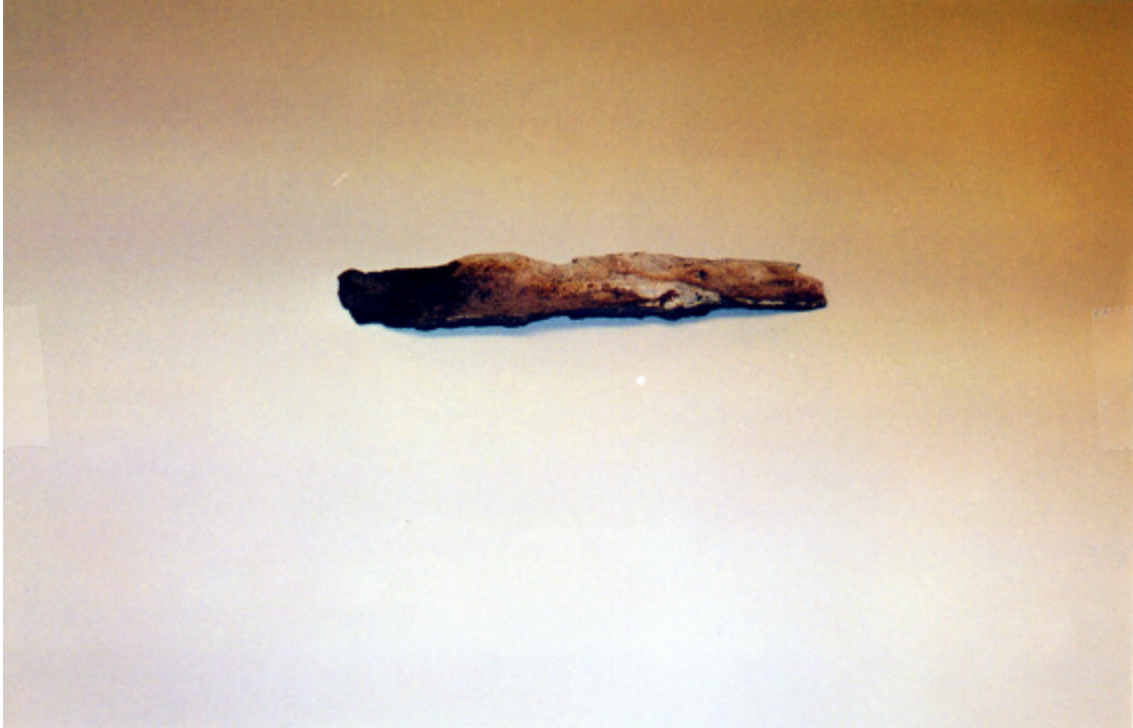
Photo #26: Flake of epoxy grout from 66" intake pipe - (5" x 1/16").
