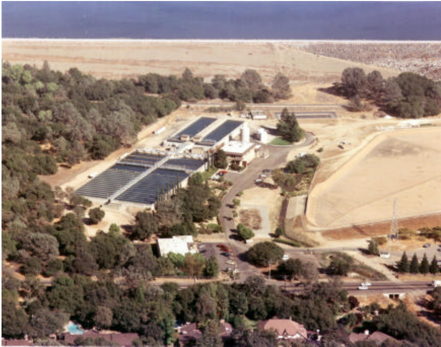
San Juan Water District Water Treatment Plant. Pretreatment basins are in foreground, filter basins are in background, with a portion of Hinkle Reservoir on the right of the photograph.
