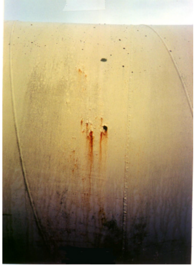
Photo #5: Exterior coating deterioration and pitting typical of many areas of 42" intake pipeline.
