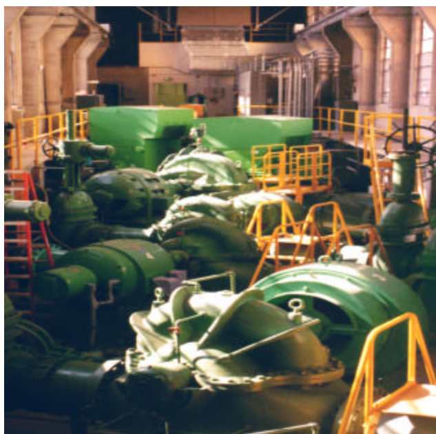
Folsom Pumping Plant
