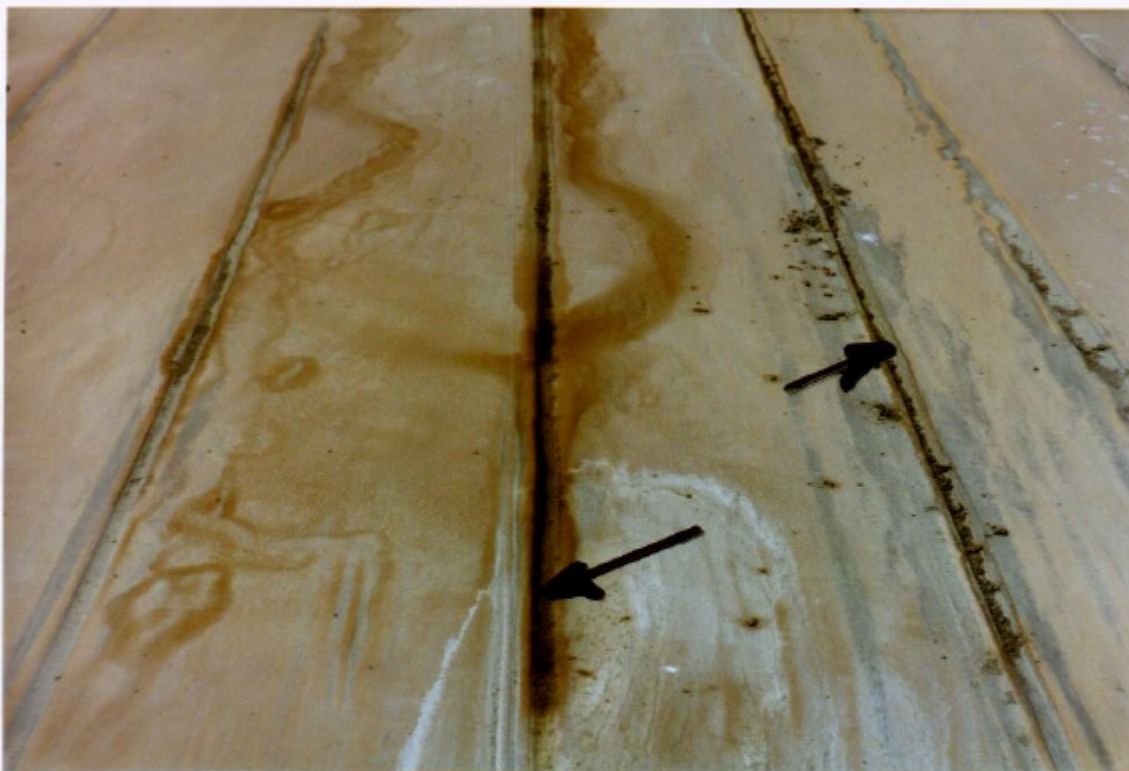
Figure 14. Photo Illustrating Debris in Factory Seam Area as well as Dark Brown Discoloration.
