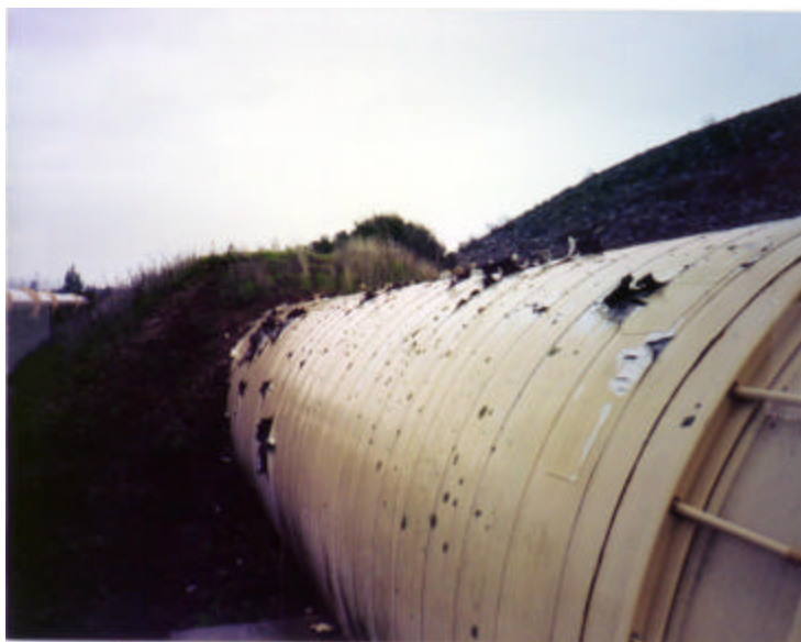
Failing Exterior Tape Wrap
