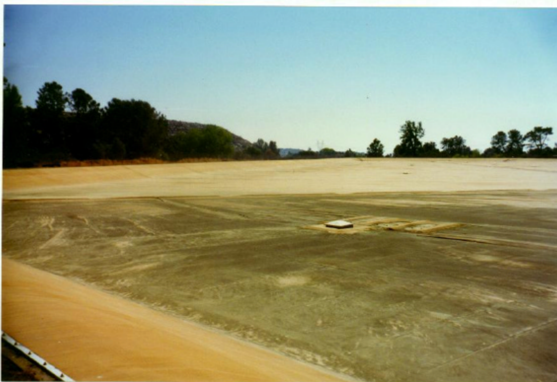
Figure 2. General View of Hypalon Cover Taken from the North. Note the Dark Grey Discoloration of the Surface.
