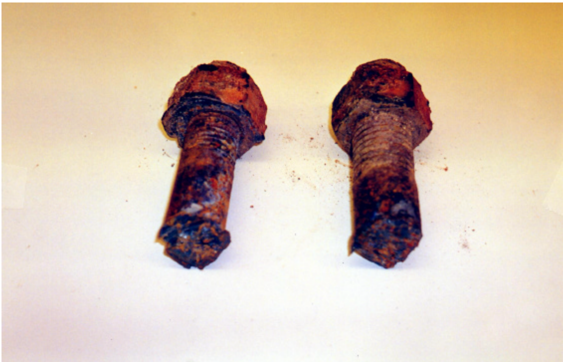
Photo #27: Rusted 1 1/4" steel bolts cut from 42" pipeline access manhole.
