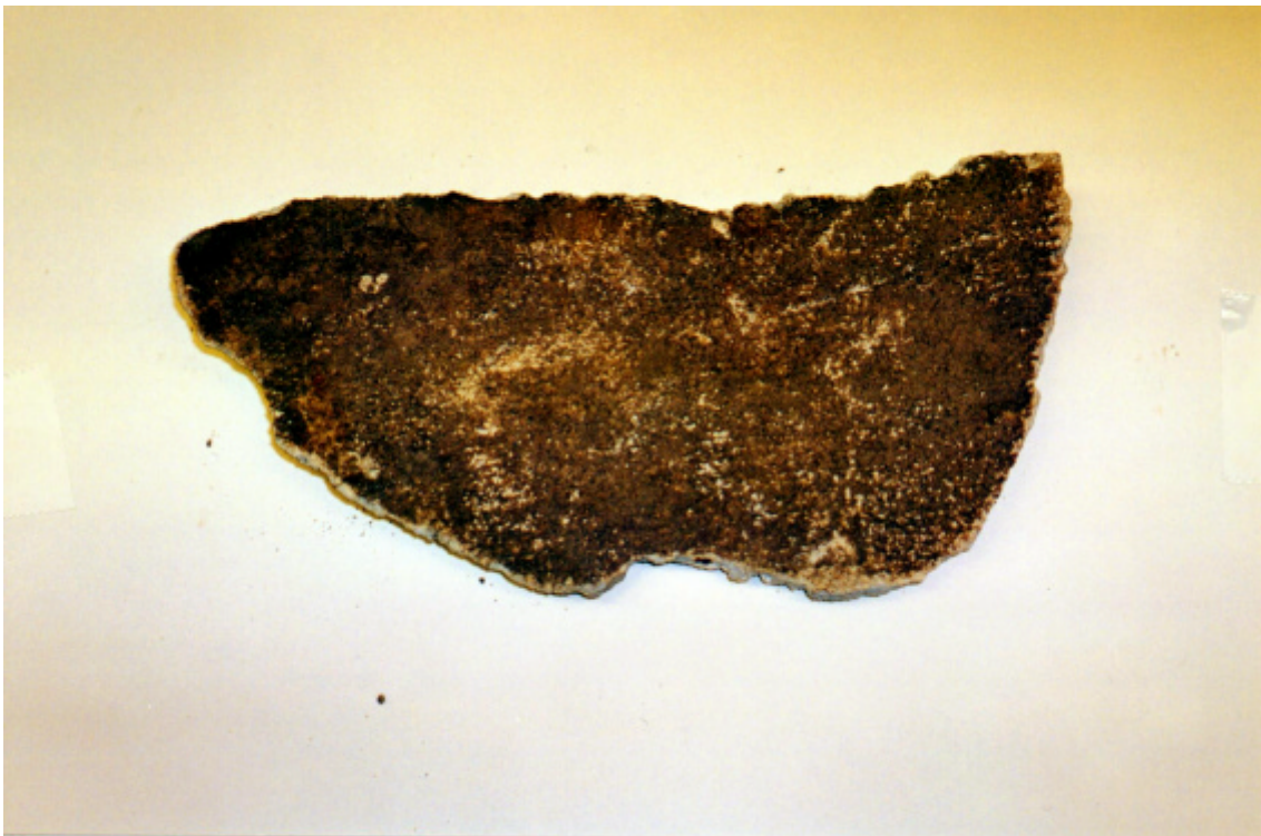
Photo #25: Loose chunk of 1/2" cement lining (8" x 5") found lying on bottom of 66" P.L..
