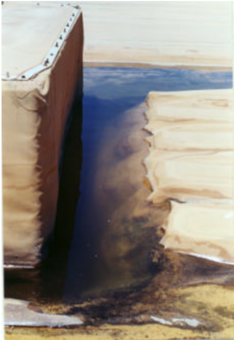
The Hypalon cover at the outlet structure should be redesigned to eliminate the undrained sump.
