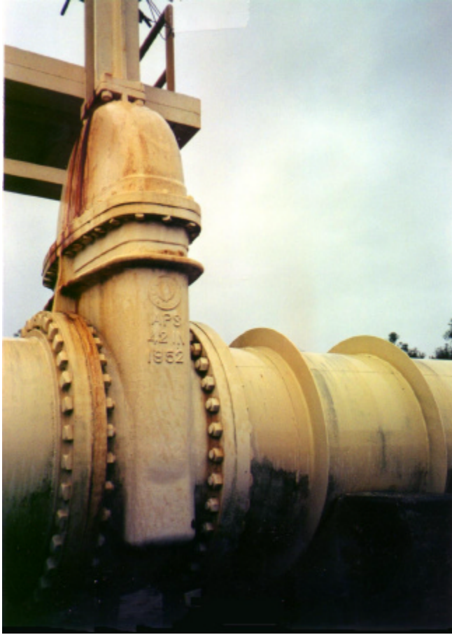
Photo #4: 42" Gate valve on intake pipeline near 84" USBR P.L.
