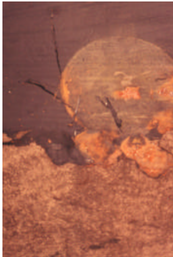
Corrosion Present under Failed Coal Tar Lining
