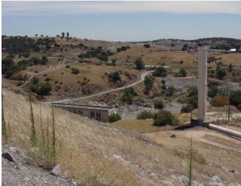
Bureau's Raw Water pipeline. The Bureau's Folsom Pumping Plant is shown near the center of the photograph. The first surge tower and a portion of the 84-inch pipeline are on the right. The raw water pipeline serving the City of Folsom can be seen in the background.
