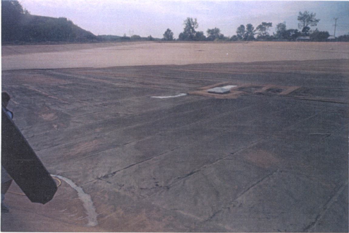
Figure 3. Photo showing the discolored cover area due to standing water - NE quadrant near inlet
