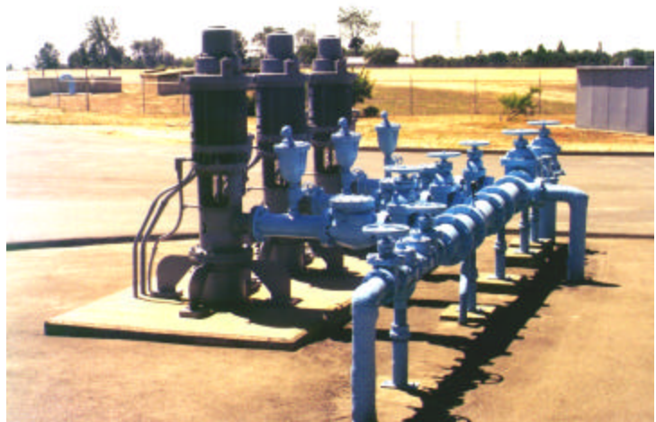
The in-plant pump station should be replaced with a properly designed side-stream pump station.
