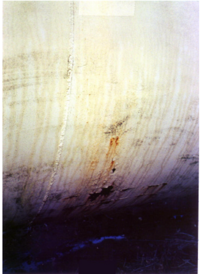
Photo #2: Corrosion, deterioration, and pitting on surface of 72" P.L. about 50 feet from USBR turnout.
