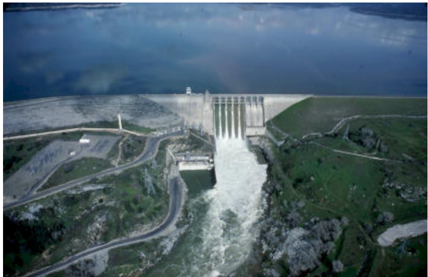
Folsom Dam. Bureau’s Pumping Plant and 84-inch Transmission Pipeline are shown near the base and to the left of the dam.
