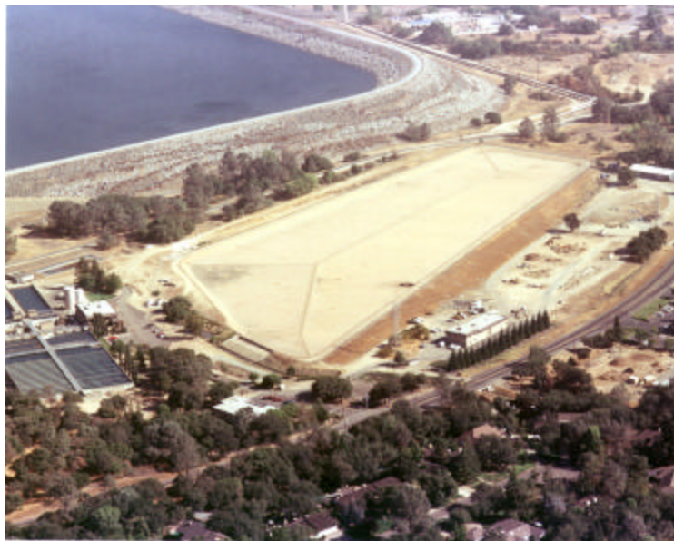
Hinkle Reservoir. The District's WTP can be seen to the left. A portion of the Bureau's 84-inch pipeline and one standpipe can be seen at the top of the photograph.
