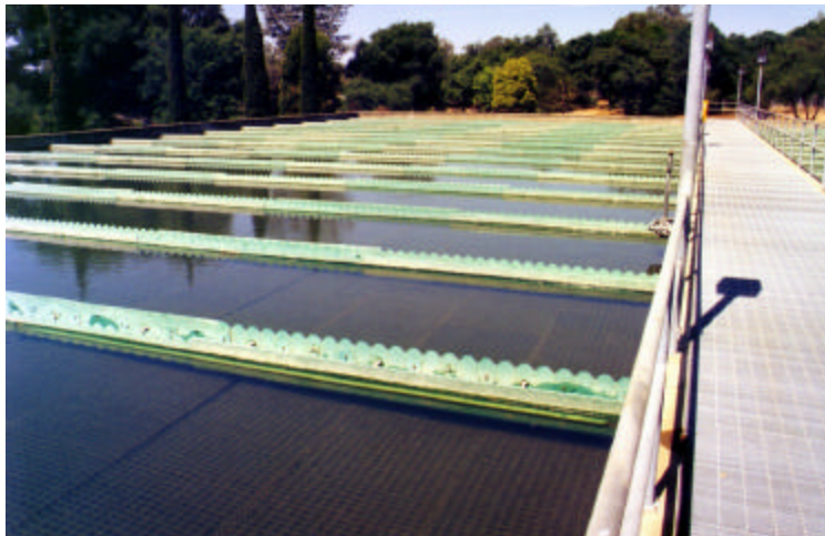
The sedimentation basin launders and the settled water channel are examples of existing WTP hydraulic elements that will require significant improvements.
