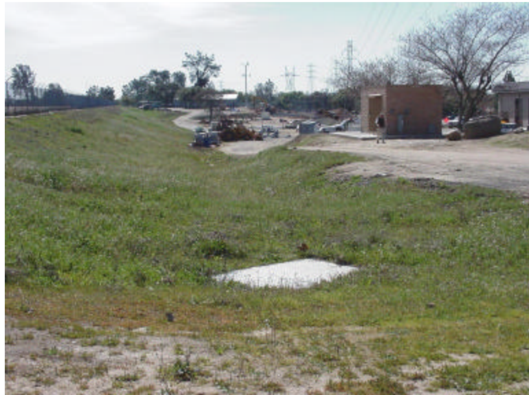
View down west side of reservoir. Existing 48-inch bypass is located between toe of reservoir berm and pump station shown on right.
