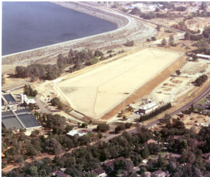
Hinkle Reservoir. The District's WTP can be seen to the left. Folsom Reservoir is at the top left of the photograph.
