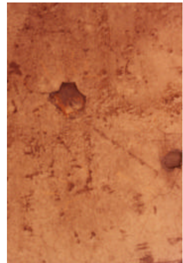
Cracked and Failed Coal Tar Lining
