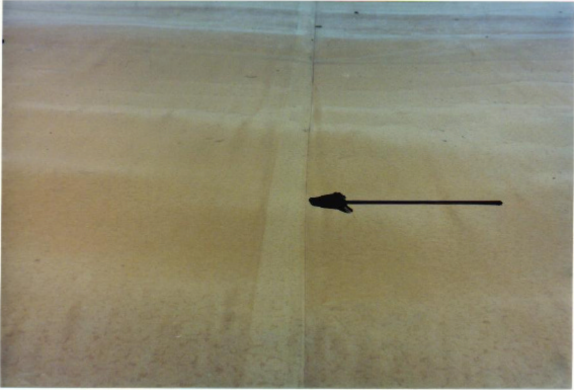
Figure 5. Photo Showing Typical Factory Fabrication Seam.
