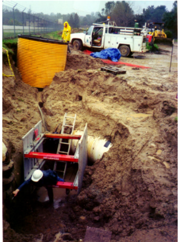
Photo #8: 42" Wye pipe, butterfly valve and tape wrap coating at Location 1.
