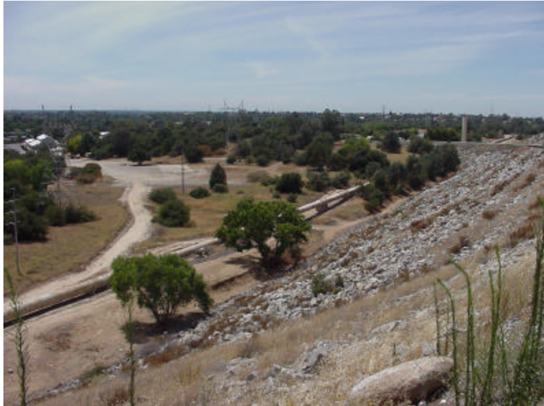
Bureau's 84-inch pipeline. Location is near Folsom dam, at base of dam road. Second surge tower can be seen in background.
