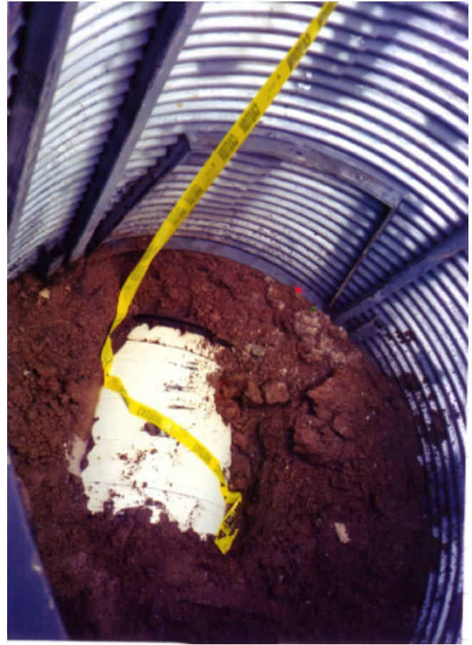
Photo #11: Tape wrap on 42" P.L. at Location 2 with \frac{3}{4} " of tape delaminated at FCA.
