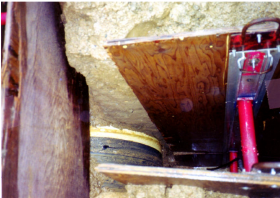
Photo #12: Diaper on joint of 66" CLS pipe at Location 2.
