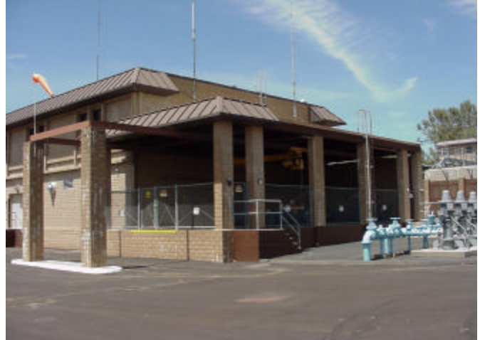
The chlorine area will need to be enclosed and provided with a scrubber to comply with current safety requirements.
