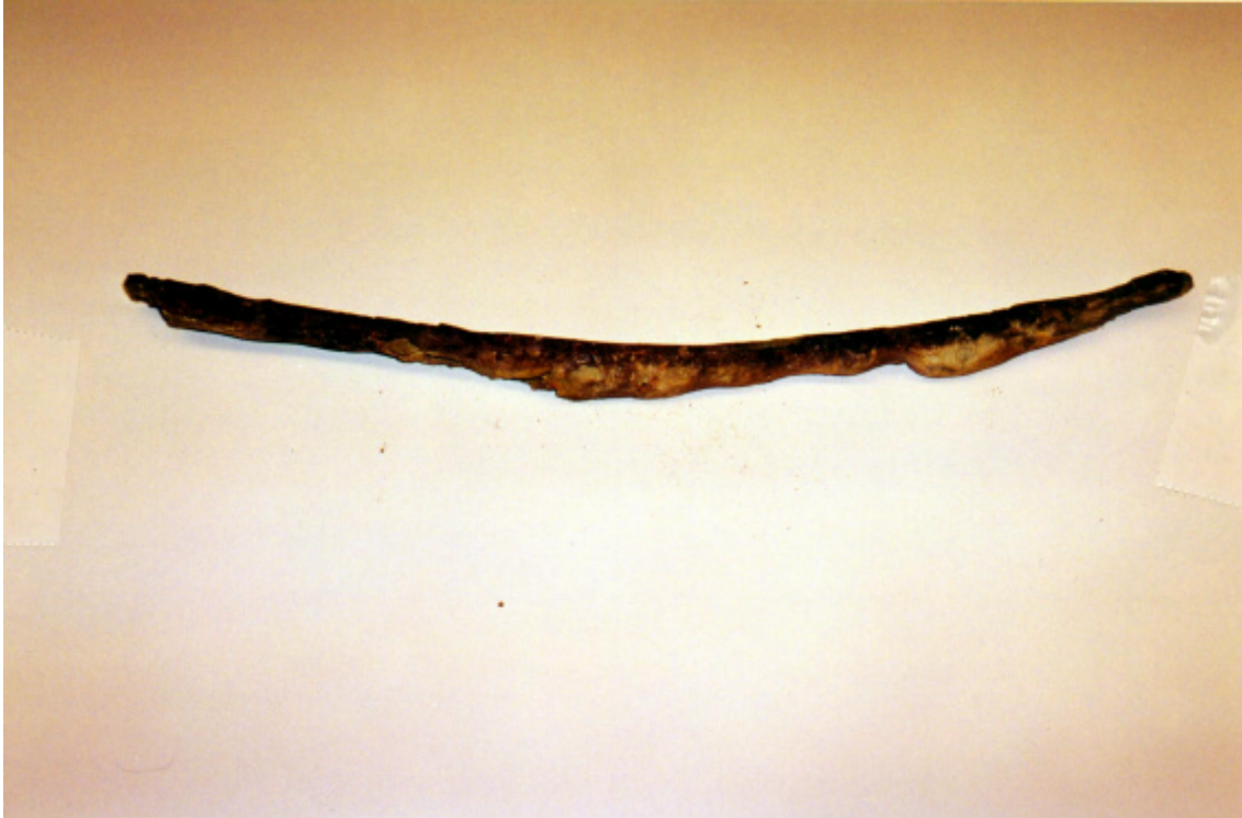
Photo #24: Chunk of grout which fell away from interior joint of 42" P.L. (16" x 1").
