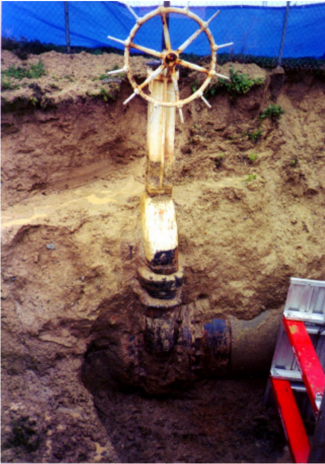
Photo #10: 54" gate valve south of Location 1, 54" CMC Steel with epoxy at FCA, gate valve protected with tape wrap and coal tar.
