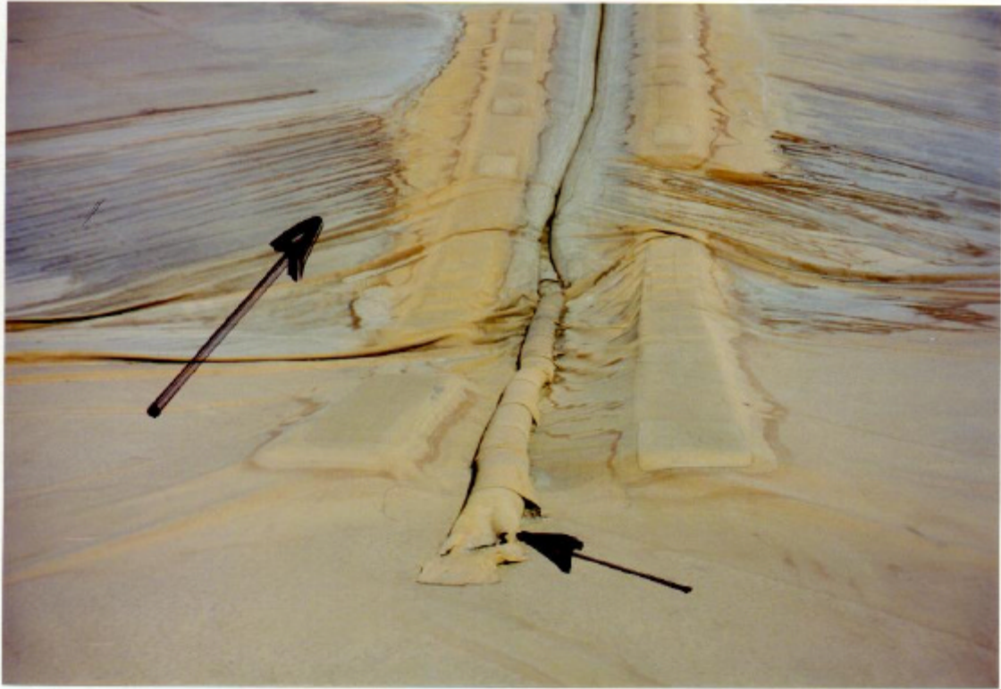
Figure 11. Photo Illustrating Sand Ballast Tube Damage and Cover Wrinkling - South End of Reservoir at Slope.
