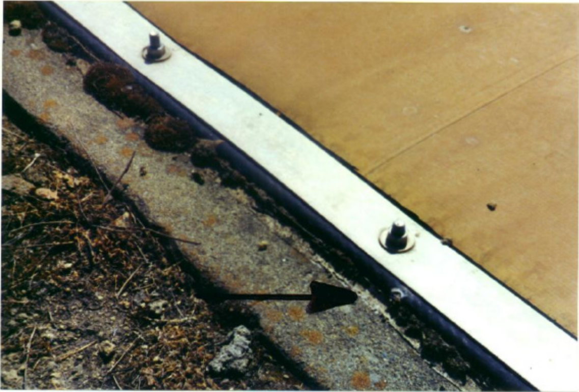
Figure 3. Typical Top of Slope Batten Bar Connection Detail. Note Deteriorating Condition of Edge Seal.
