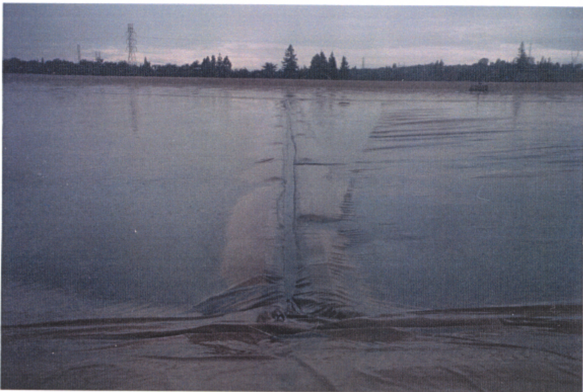
Figure 4. Photo showing poor surface drainage into the sump - NE sump
