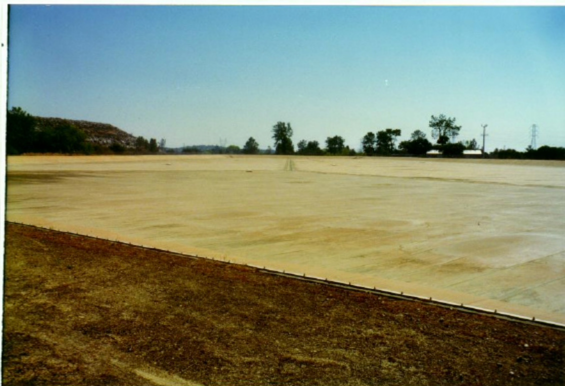
Figure 1. General View of Hypalon Floating Cover - Note Tensioned Condition
