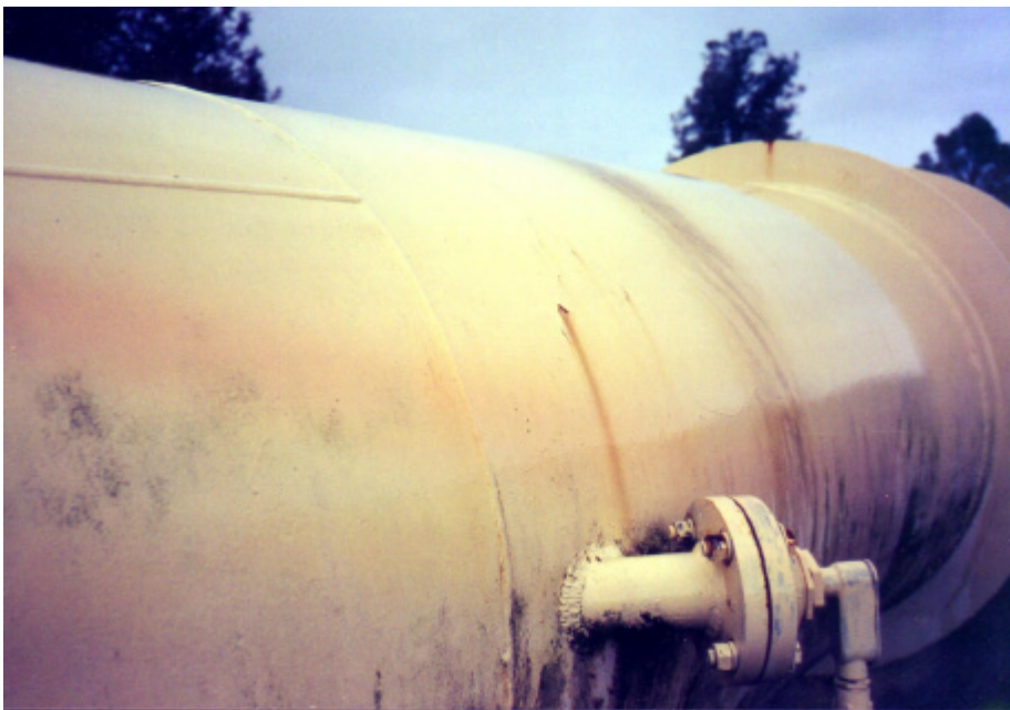
Photo #6: Corrosion pits near 42" Venturi section of intake pipeline.
