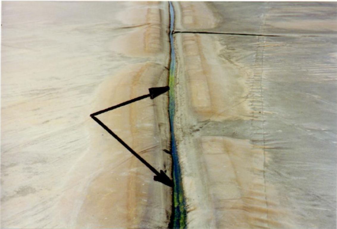
Figure 12. Rainwater Collection Sump With Algae Growth - NE Corner.
