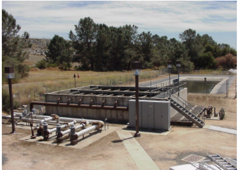
The existing backwash water recovery system should be demolished and replaced with a new, properly sized, reliable system.
