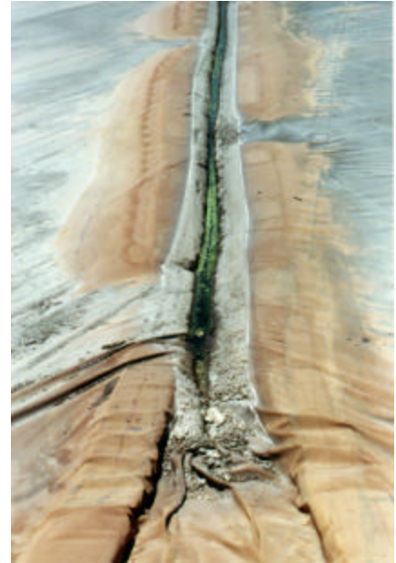
Sumps within the Hinkle Reservoir cover should be cleaned of all debris and algae.
