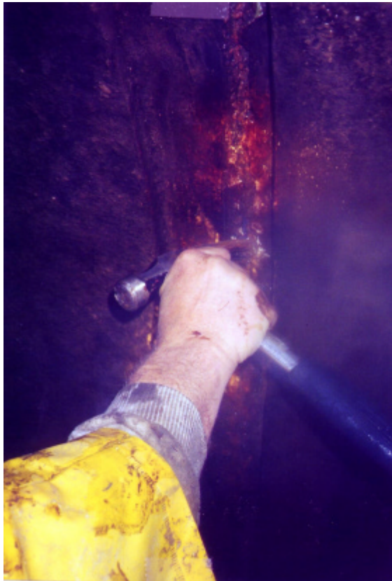
Photo #19: Deteriorated epoxy grout in joint and rust in interior of 72" P.L.
