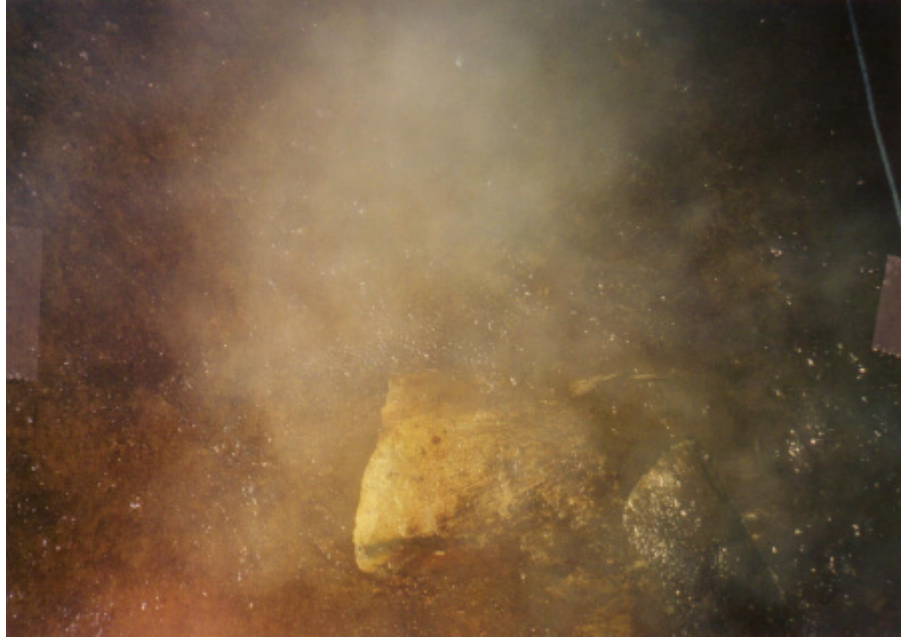
Photo #22: A chunk of concrete lining in bottom of 66" P.L. north of Location 1.
