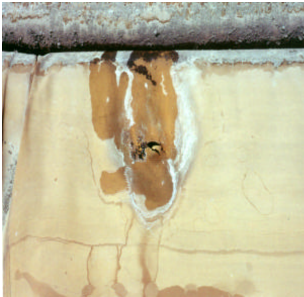
All holes and failing patches should be repaired.
