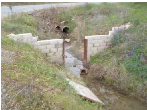
Figure 1: Existing Solar Field Culvert
