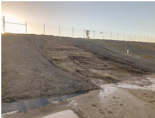
Figure 1 Hinkle Reservoir Embankment
