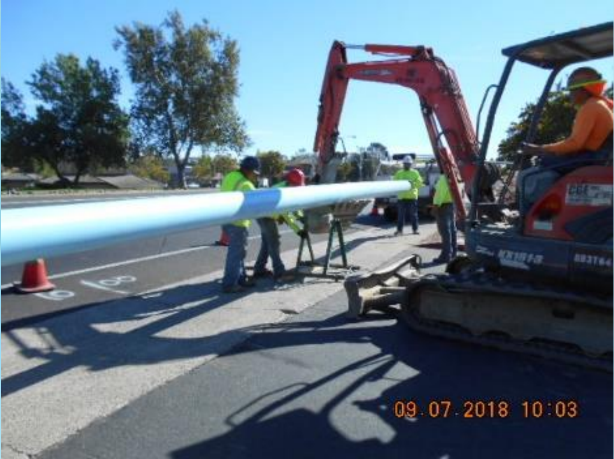
Pipe Ready for Insertion
