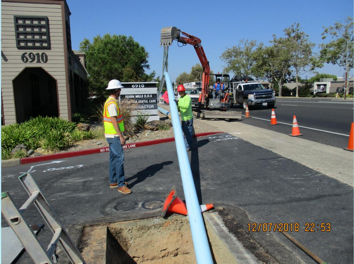
Fused Pipe Being Inserted
