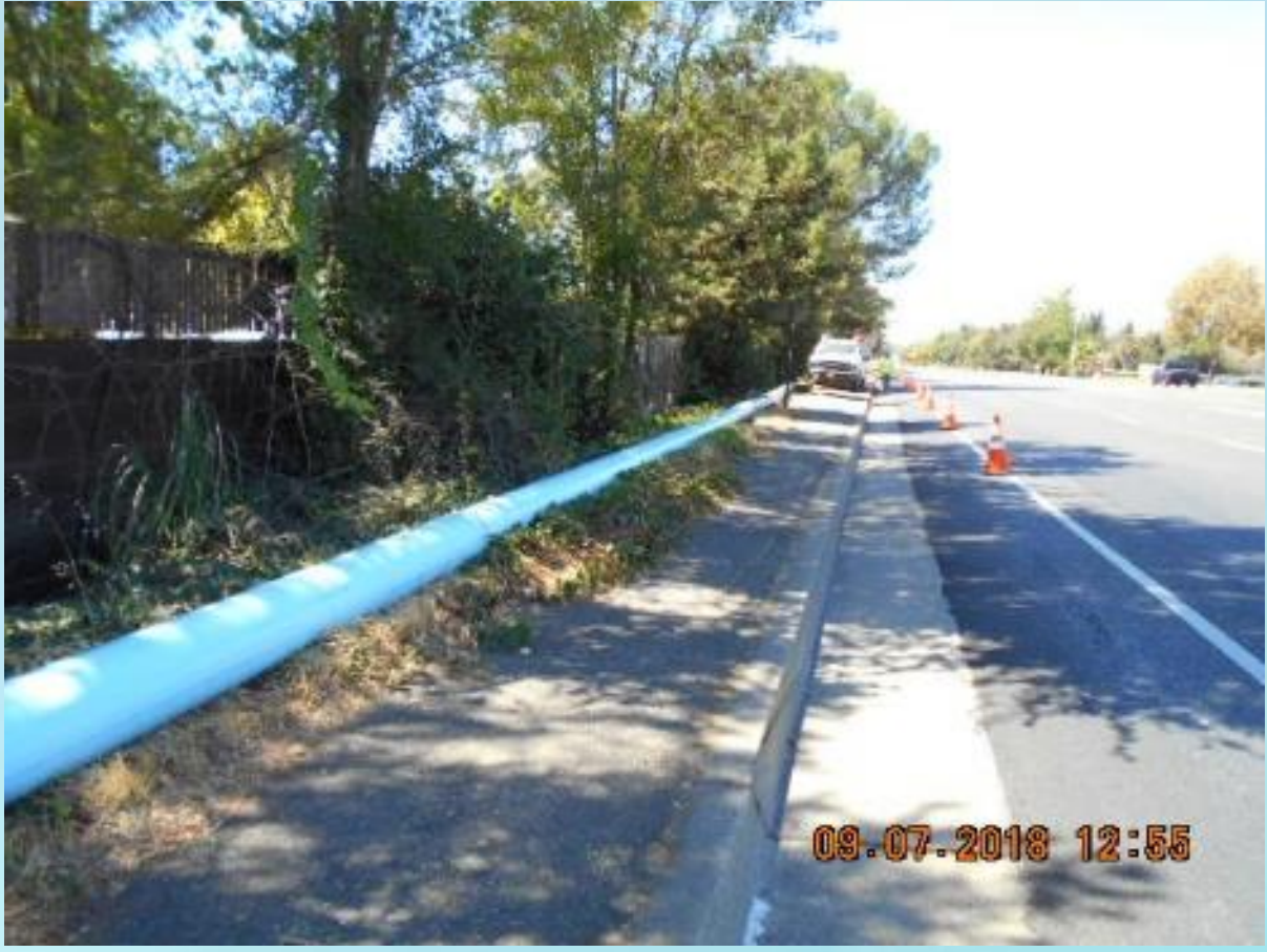
Fused Pipe Ready for Insertion
