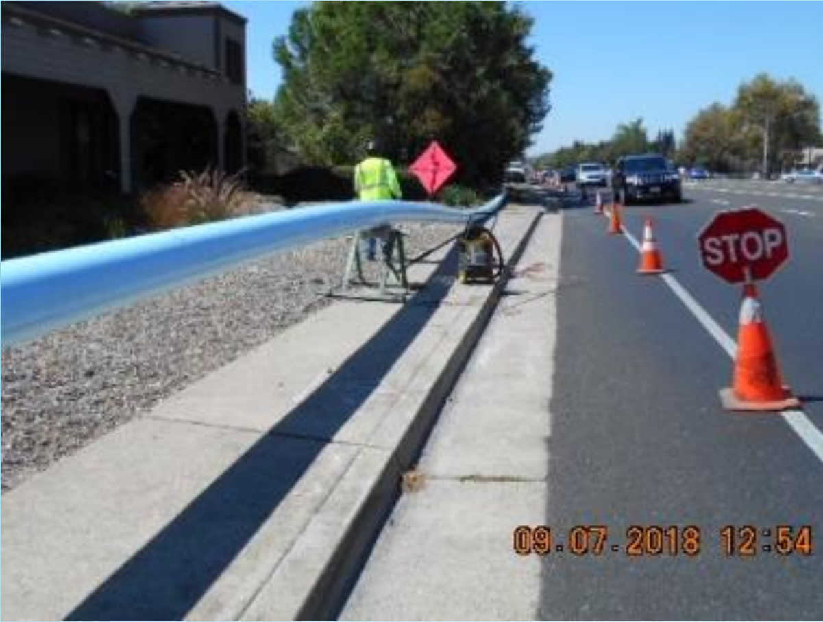
Pipe Fusing Operation
